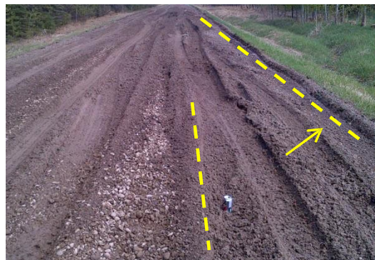
Fig. 2 Mountain View County Road damage caused by drilling rig move – rutting and road edge pushed out
