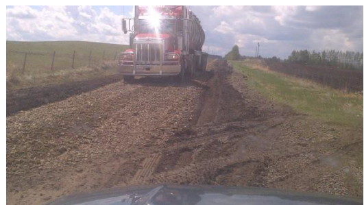
Fig. 6 Mountain View County Damage has required operator to lay pit run gravel in the centre to allow continued movement of trucks
